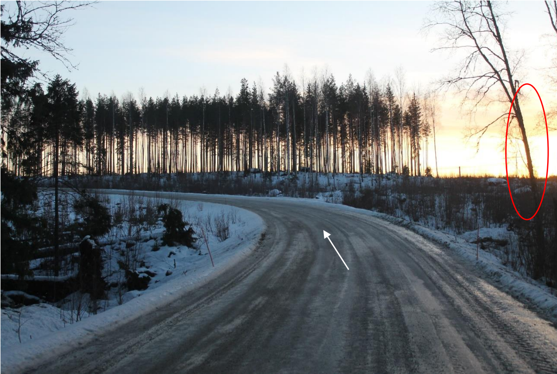
Pos 26/Pic 7. Road 2492. https://maps.app.goo.gl/mRQHmcV67FBDLQV26 Marked tree need to cut on private property.
