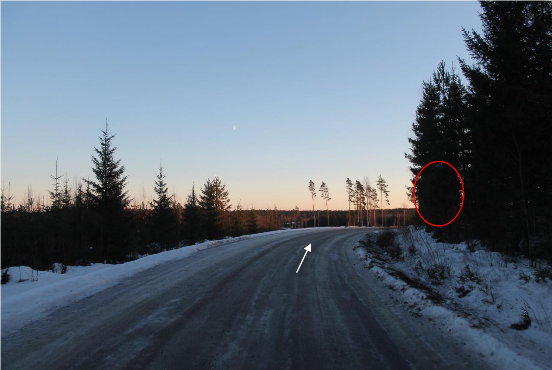
Pos 20/Pic 5. Road 2492. https://maps.app.goo.gl/rwKitBoPhSPJTwvd6 Marked trees need to cut.
