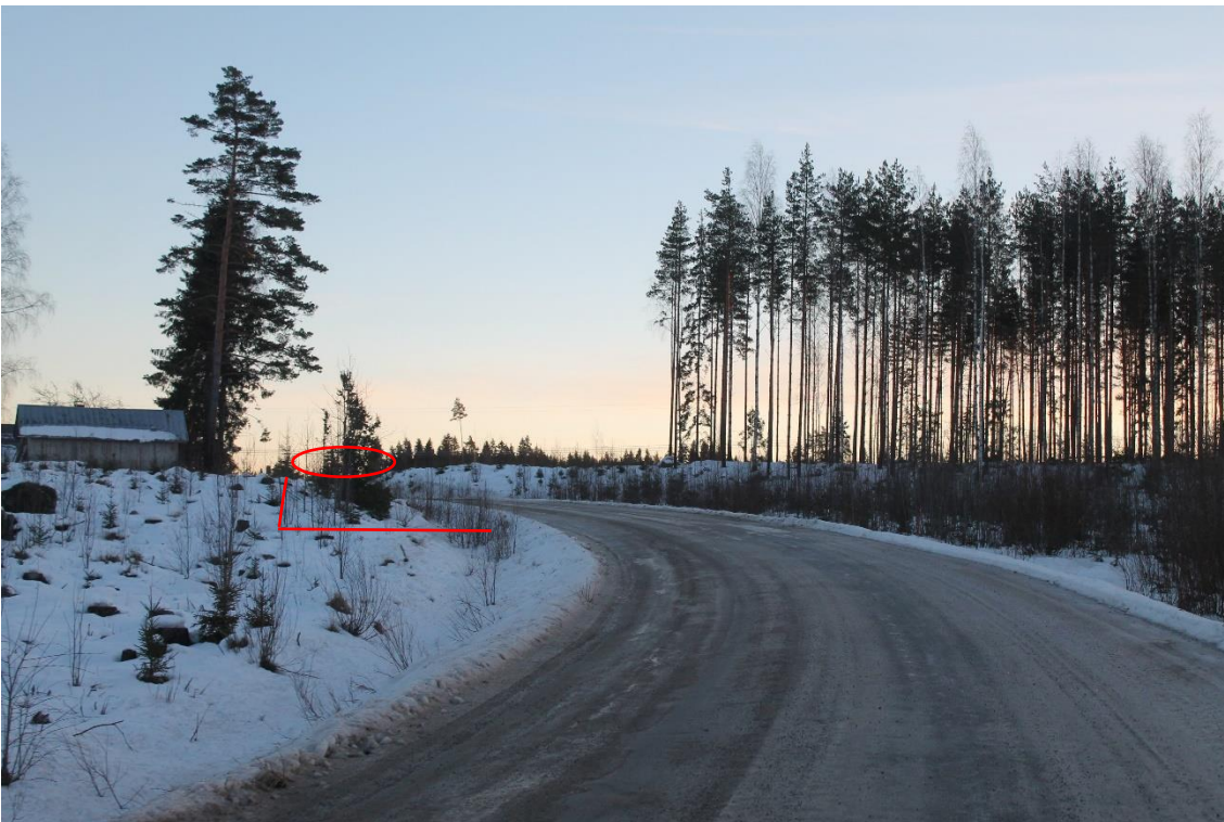
Pos 26/Pic 8. Road 2492. https://maps.app.goo.gl/mRQHmcV67FBDLQV26 Marked trees need to cut on private property. Marked area need to be flat.
