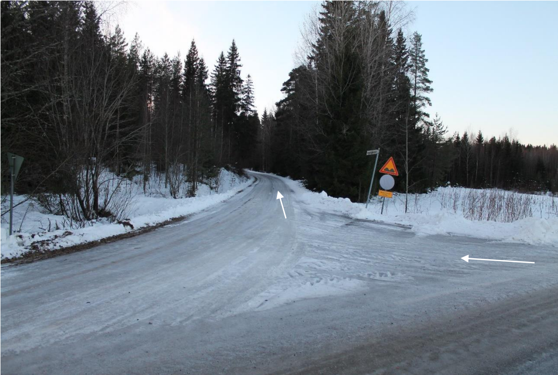
Pos 29/Pic 11. Turning from road 2492 toward Vuohijoentie. https://maps.app.goo.gl/Wyz1T9j6cdKAwRt37 Site entrance to be build according to specifications for site roads.
